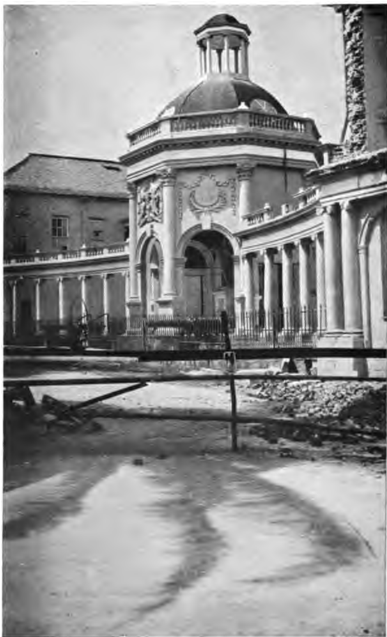
RODNEY'S MONUMENT, SPANISH TOWN. The damage done by the earthquake will be noticed.
